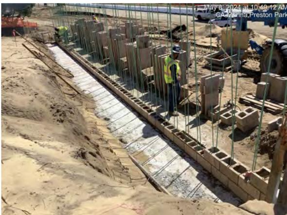
Installing concrete blocks for sound wall near Preston Park
