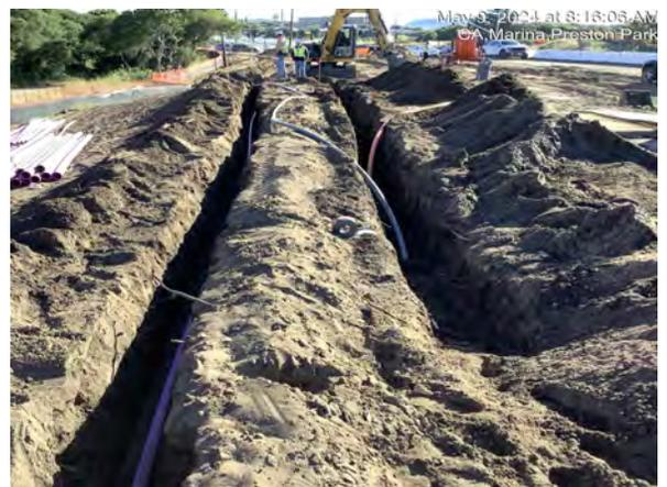
Trenching/installing irrigation service lines near Preston Park
