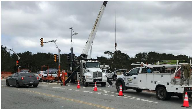
Removal of Abrams existing signal poles and placement of temporary signal poles
