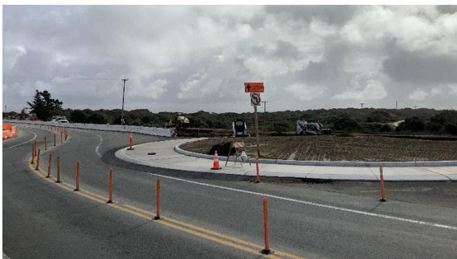
Earthwork and grading for the Preston roundabout median
