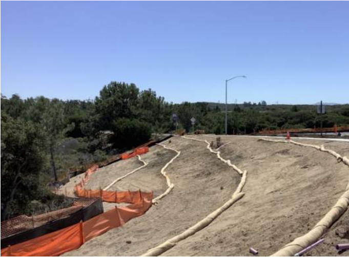
Installing straw waddles for erosion control on side slopes at Abrams Drive
