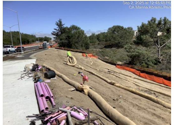
Installing straw waddles for erosion control on side slopes at Abrams Drive
