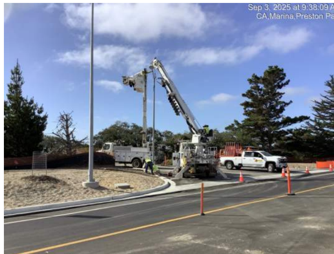
Removing old street light pole at Chapin driveway
