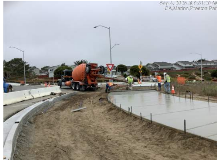
Placing concrete for curb & gutter and sidewalk at Preston Drive
