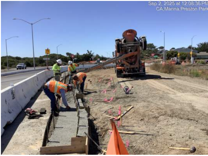
Placing concrete for curb & gutter and sidewalk at Preston Drive
