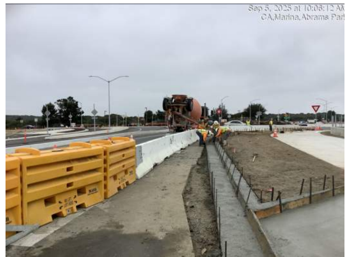
Placing concrete for curb & gutter and sidewalk at Abrams Drive
