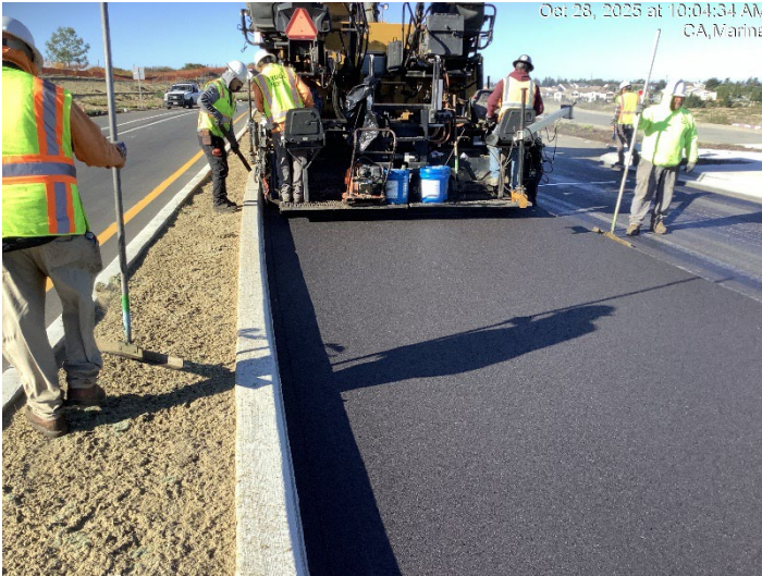
Paving final lift for WB direction
