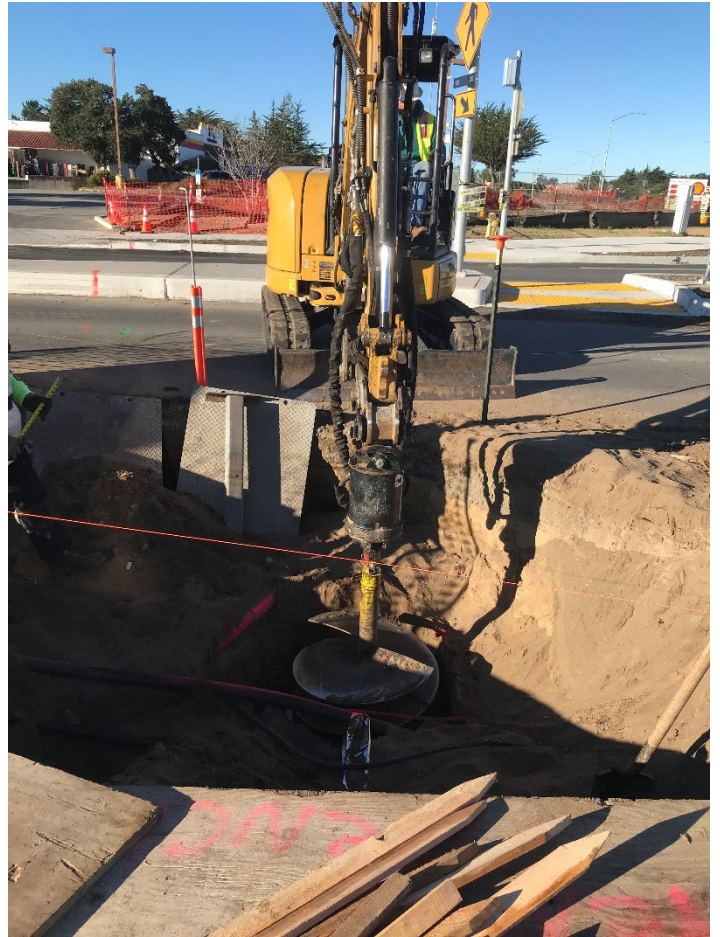
Placing the last street light foundation now that PG&E has relocated underground utilities
