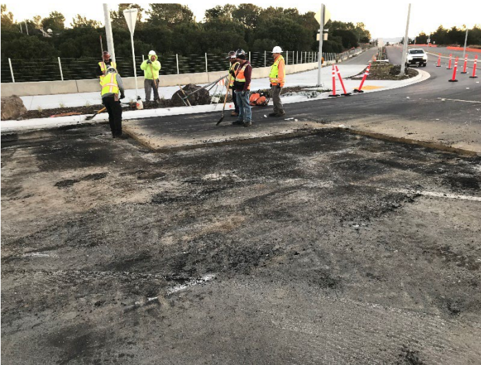
Conforming another day of paving the final lift to the previous day
