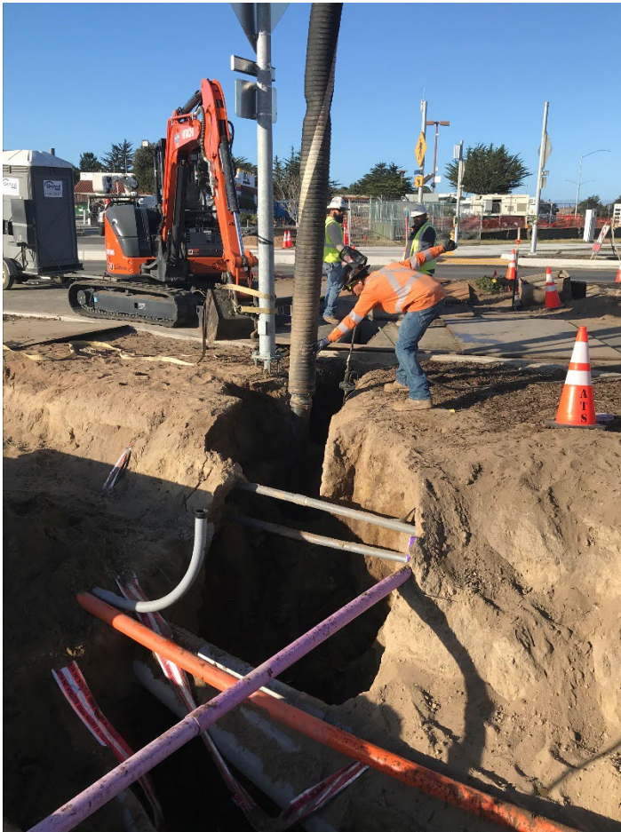
PG&E utility relocation work
