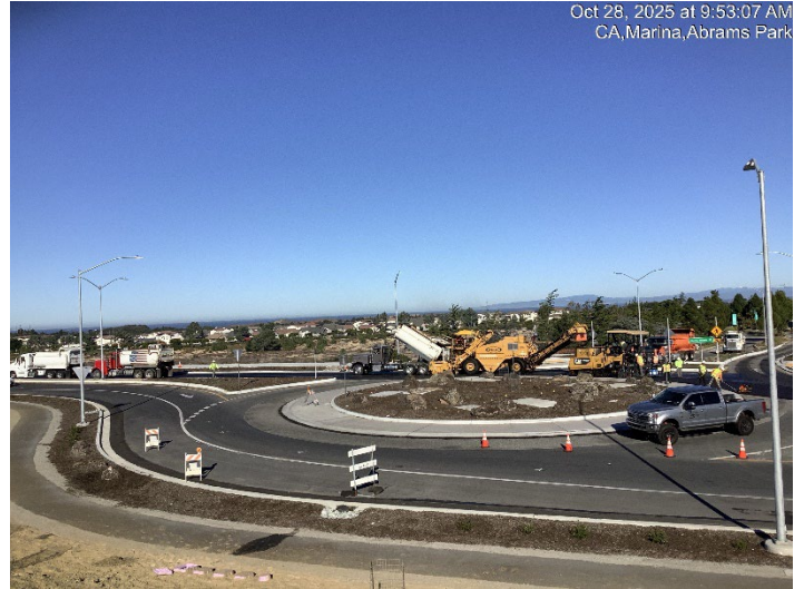
Paving final lift for WB direction
