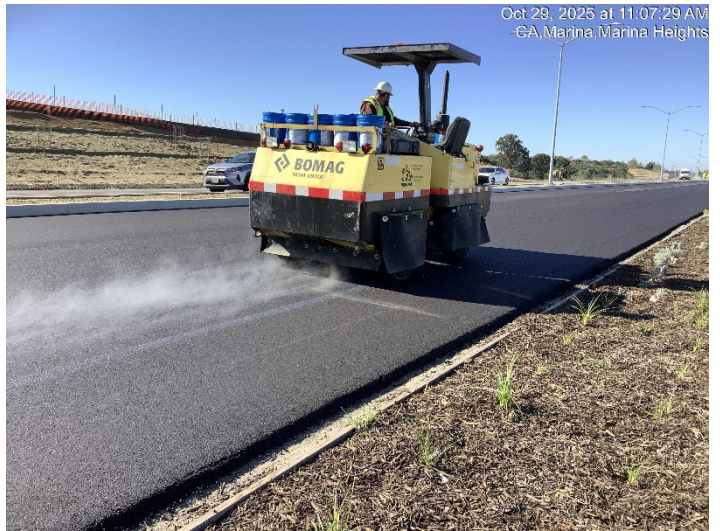
Rolling final lift for compaction
